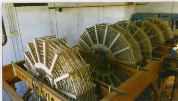
Photo 5: Inside the Woodbrook Coil House showing the impressive tuning coils in their timber mounting rack.
