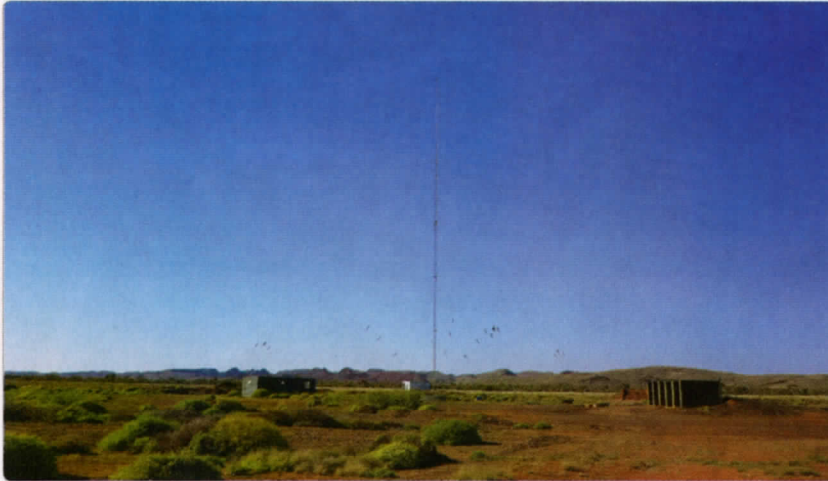
Photo 1: The Woodbrook antenna and station.
