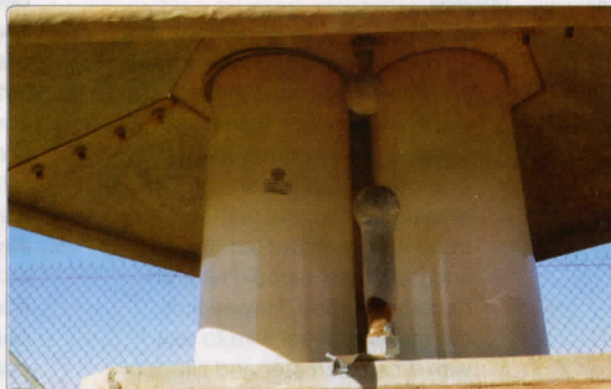
Photo 2: The porcelain insulators at the tower base, together with a spark gap for static discharge and lightning protection.
