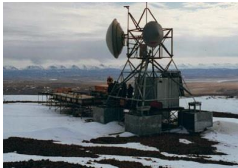
One of six repeater microwave stations connecting CFS Alert and Fort Eureka.
