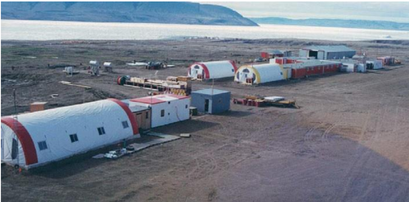
Fort Eureka, Ellesmere Island, NWT, 500 kilometres south of CFS Alert.
