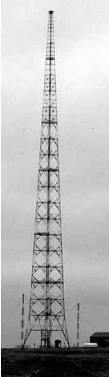
Fig. 12. The 633-foot self-supporting tower at Cambridge Bay. (Author’s collection, credit Judith Banning)
