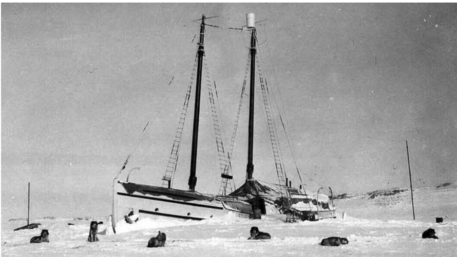
Fig. 10. Antennas on the St. Roch in the ice at Tree River. (Source: Parks Canada St. Roch photograph collection, H5FR-30-12)
